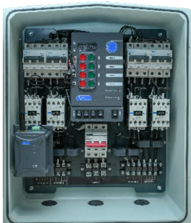
Interior View of xMU-GiA
