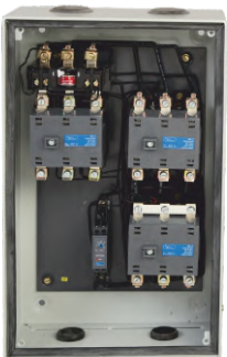
Interior View of ML FASD
