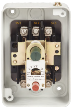
Interior View of MF1 DOL - 3Ø Starter
