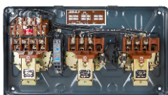
Interior View of MK2 FASD
